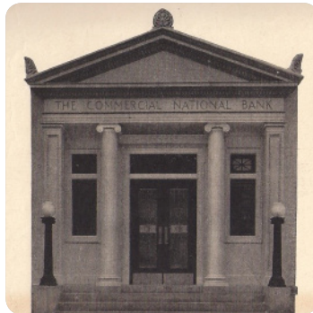
Terra-Cotta Facade 1905 79 S. Washington Street (photo 1906)
