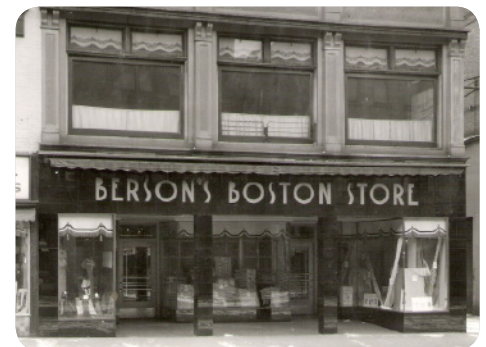
Structural Pigmented Glass Front 1935. 126-128 S. Washington St. (photo c. 1935)
