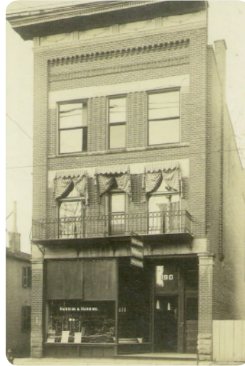
Stoner Block 1898. 190 S. Washington Street (photo c. 1910)
