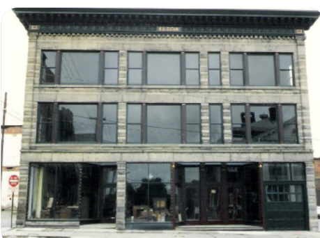
Chicago Window. Kildow Block 1898. 52-56 E. Perry Street (photo 2001)
