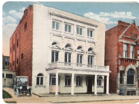
B.P.O. E. Lodge 1914 106 E. Perry Street Colonial Revival (photo c. 1920)
