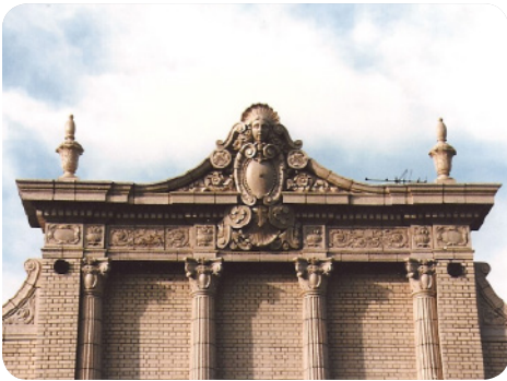
Terra-Cotta Cornice 1928. 30 S. Washington Street (photo 1984)
