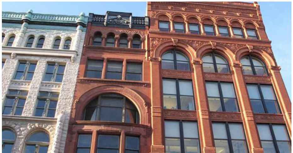
Various linear elements continue across historic facades.
