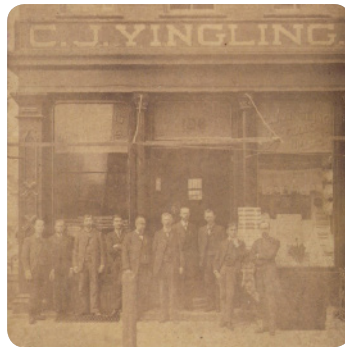
"Open Iron Front" of 144 S. Washington Street (photo 1890's)
